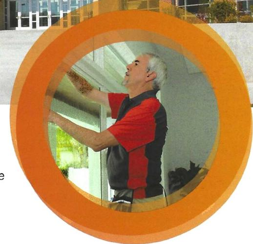
Proper installation of security film is essential to its success. For the best, most effective results the film is first adhered to the inside of the glass then a wet glaze silicone attachment system firmly secures the film and frame together. The combination of the security film and the attachment system provides additional security over a window without an attachment system.
